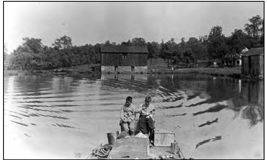
The Monocacy Basin of the C&O Canal showing the granary that was built in 1865, a building that housed a store and the Mouth of Monocacy Post Office, and a barn against the basin.
